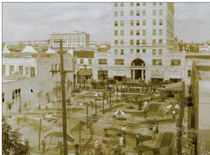
Mini-golf in West Palm Beach across from the Comeau Building on Clematis Street, 1930s. HSPBC.
