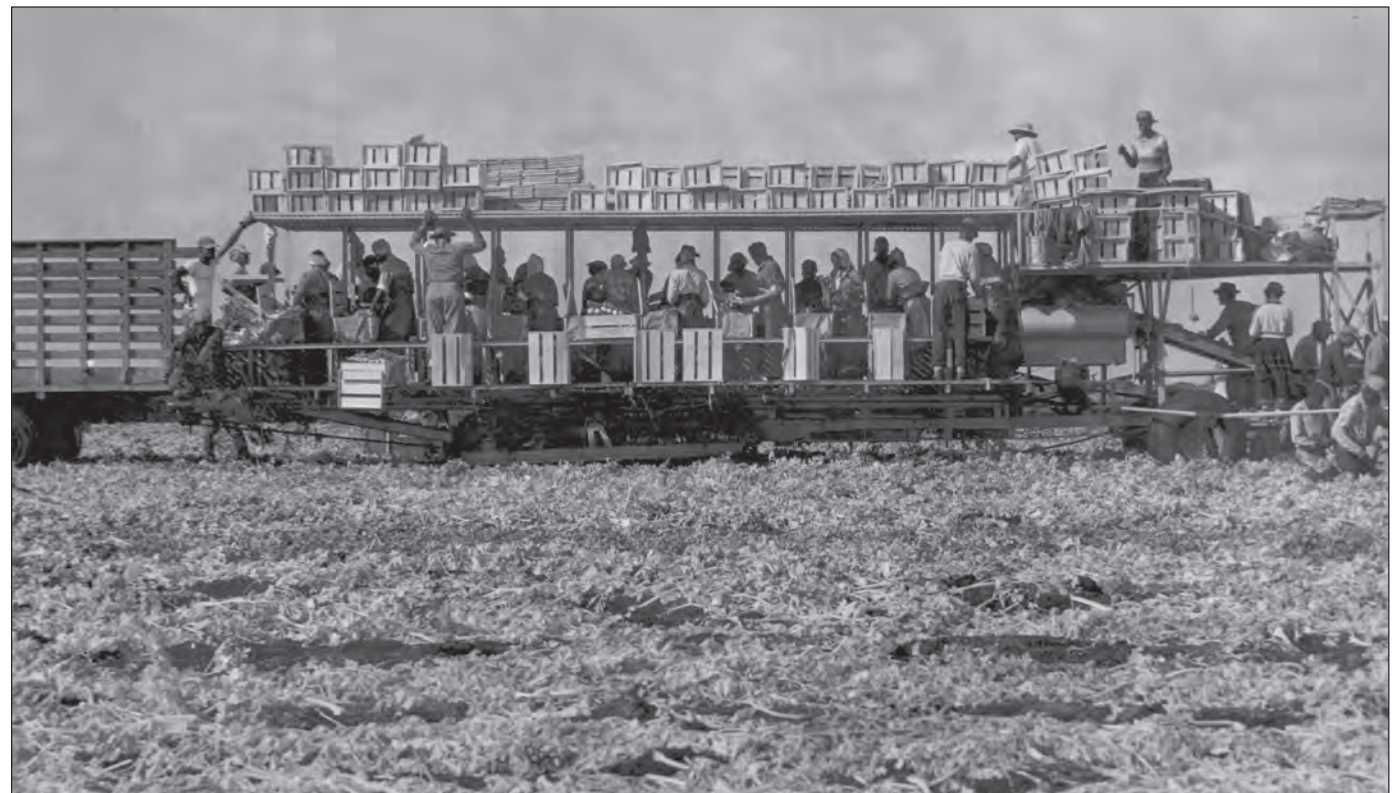
Celery harvester-packing combine used by many growers in the Everglades. Courtesy Everglades Research and Education Center.
